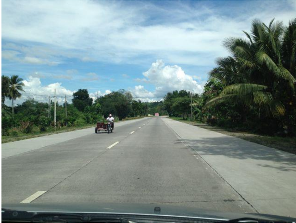
Photo 5. The national highway where part of the transmission pipeline will be laid immediately on the side of the road.
