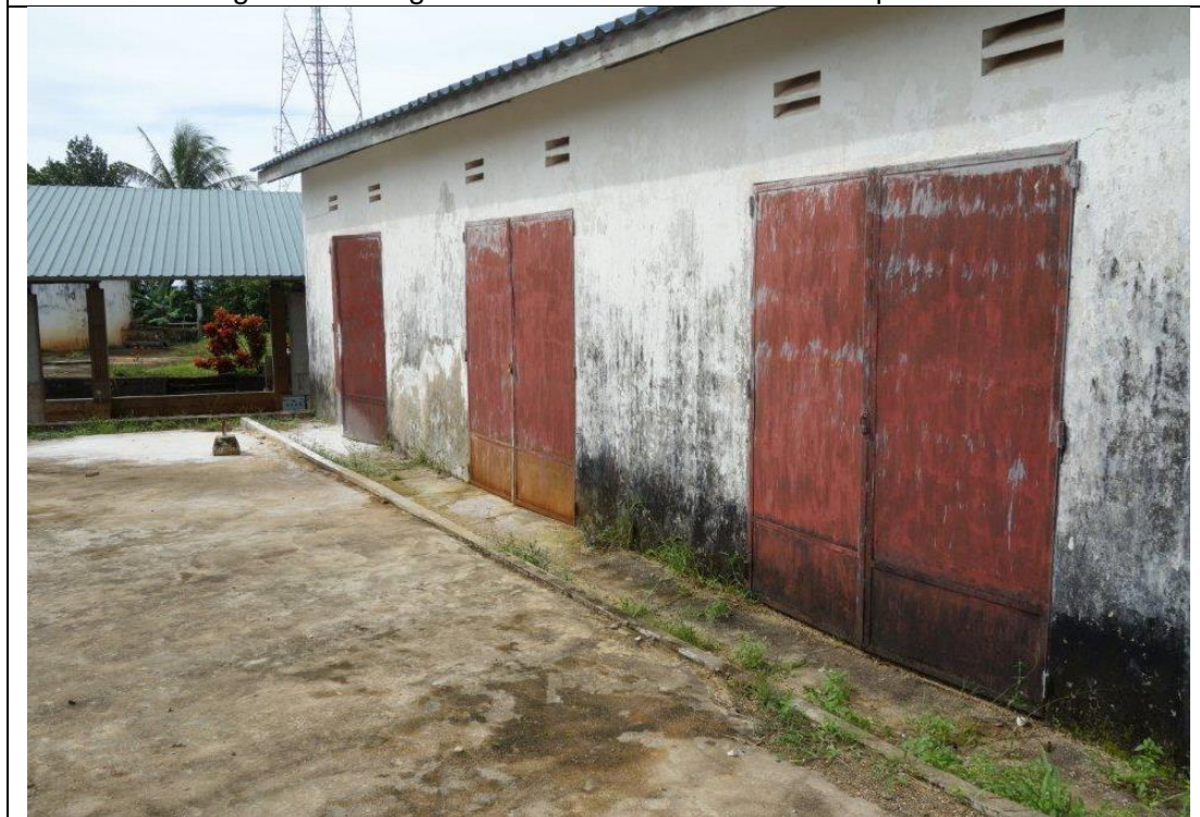
Figure 1: Storage Shed with Three Lockable Compartments
