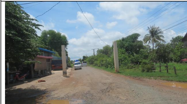
PR54 where the raw water transmission line will be laid on the road shoulder leading to the WTP.
