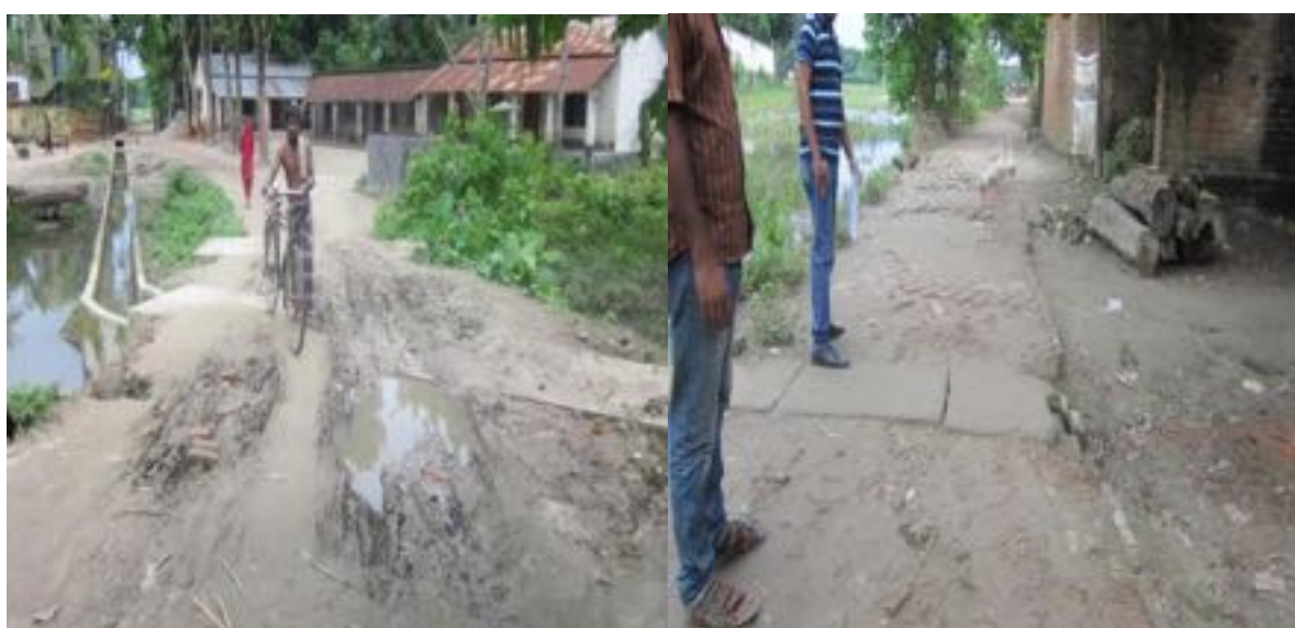
Pourashava road and drain with very badly damaged surface and displaying poor maintenance
