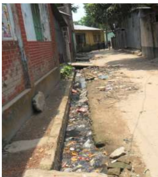
Pourashava road and drain badly damaged displaying poor maintenance
