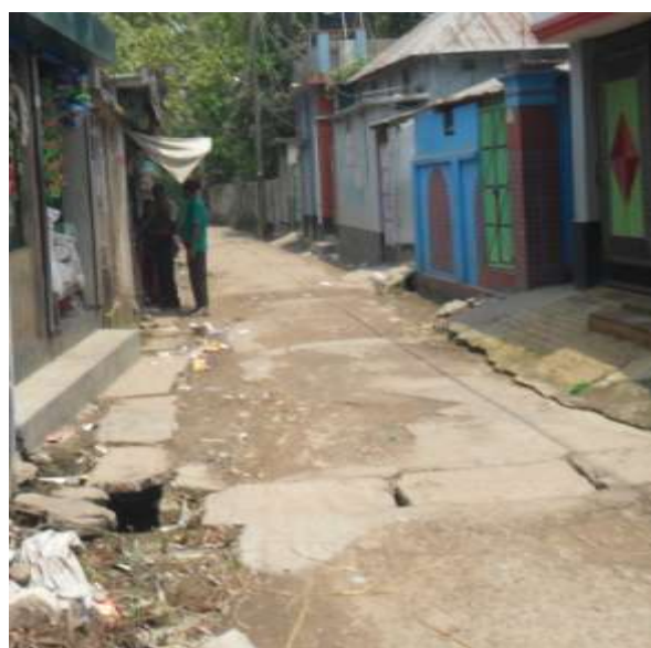
Pourashava road and drain badly damaged displaying poor maintenance
