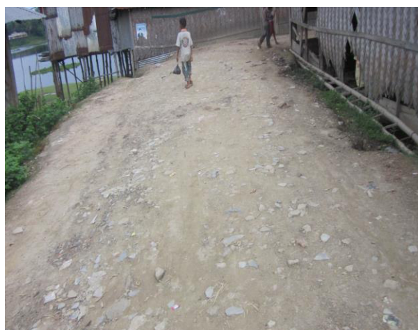
Pourashava road and drain with very badly damaged surface and displaying poor maintenance
