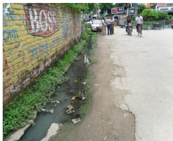
Pourashava road and drain with very badly damaged surface and displaying poor maintenance
