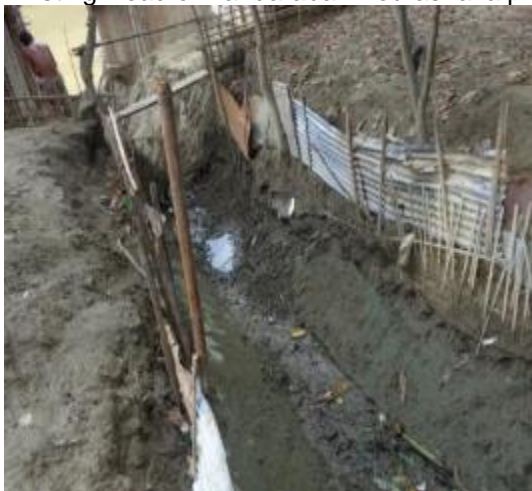
Existing Katchha Drain of Bandarban Pourashava proposed for R.C.C. drain which has a clear outfall as checked.
