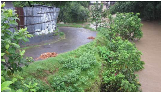
View of road PDP-14024
