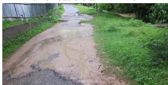
View of road PDP-14012
