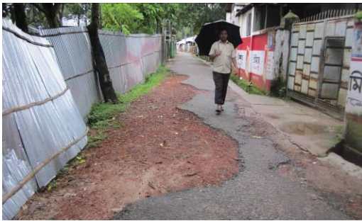
View of road PDP-14015
