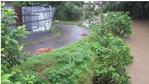
View of road PDP-14024
