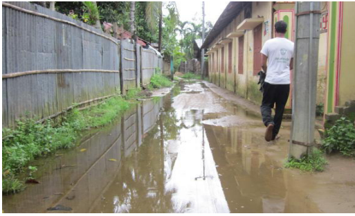
View of road & drain PDP-14017
