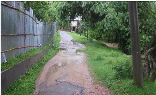
View of drain PDP-14012
