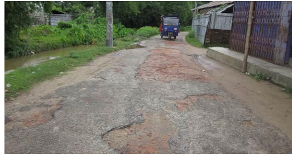
View of road & drain PDP-14011
