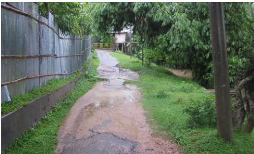
View of drain PDP-14012
