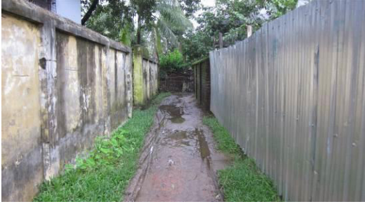
View of road PDP-14016
