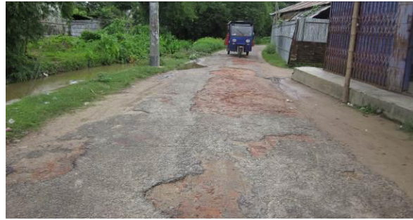
View of road & drain PDP-14011
