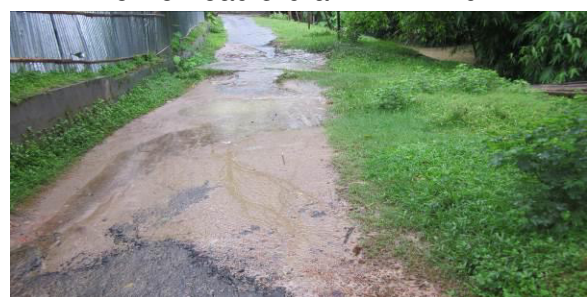
View of road PDP-14012
