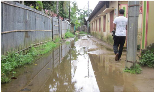
View of road & drain PDP-14017
