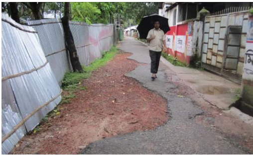
View of road PDP-14015
