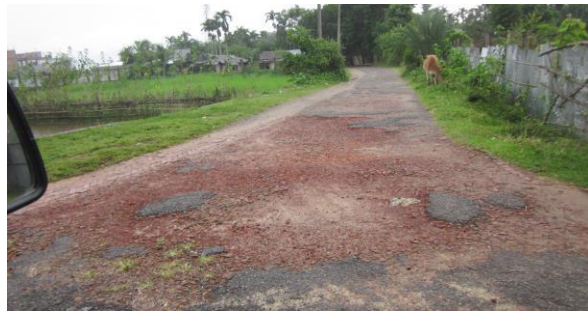
View of road PDP-14013
