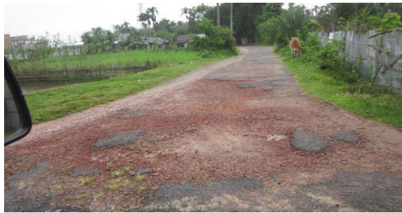
View of road PDP-14013
