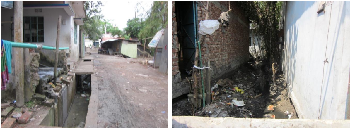
Pourashava road and drain with very badly damaged surface and displaying poor maintenance
