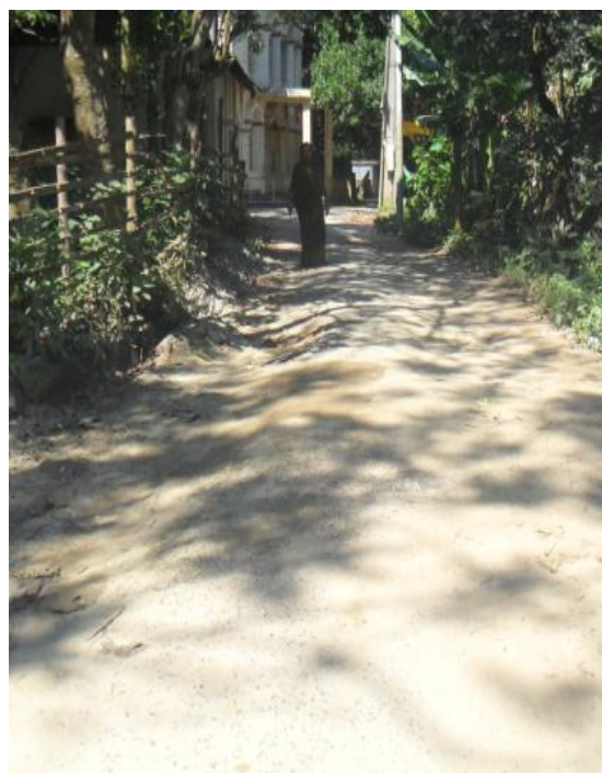
Pourashava road with badly damaged surface and displaying poor maintenance
