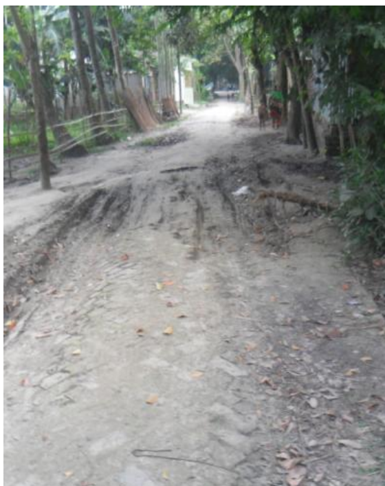
Pourashava road with badly damaged surface and displaying poor maintenance
