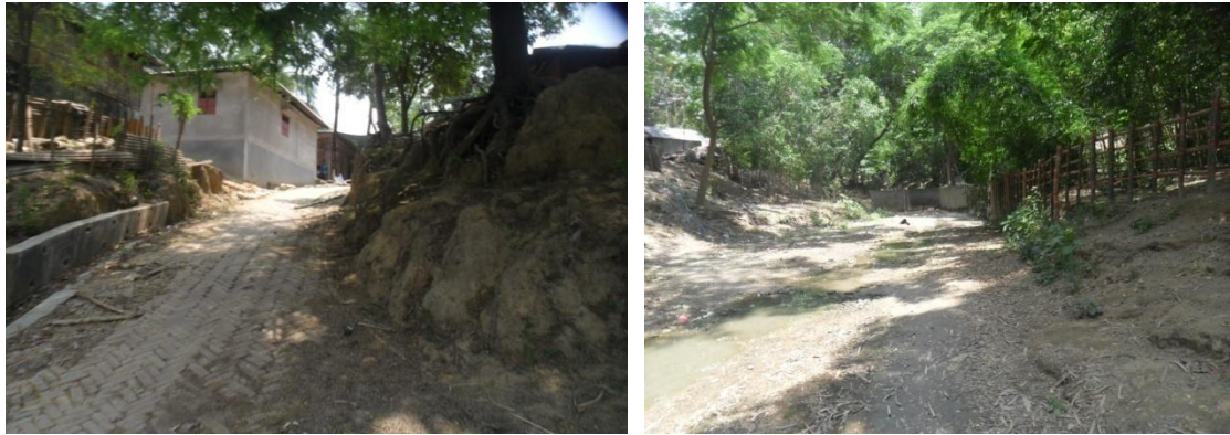
Pourashava road and drain with very badly damaged surface and displaying poor maintenance
