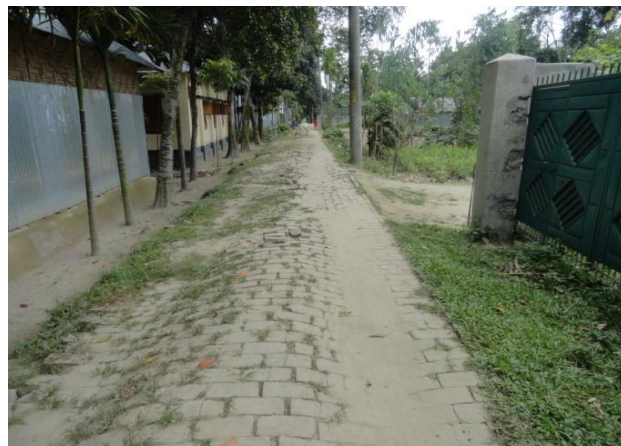
Damaged road of Panchagarh-Tetulia road of ward no. 01 (PDP 303) at Panchgarh Pourashava
