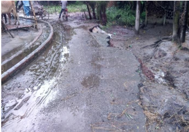
Pourashava road and drain with very badly damaged surface and displaying poor maintenance
