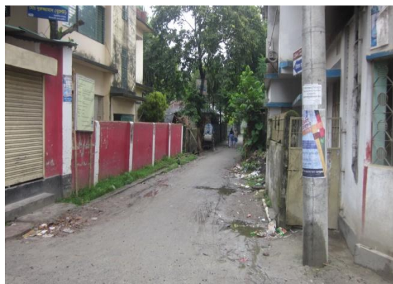
Pourashava road and drain with very badly damaged surface and displaying poor maintenance
