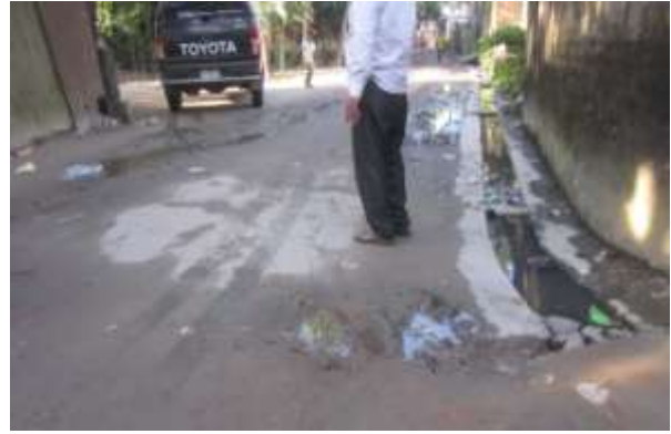
Pourashava road and drain with very badly damaged surface and displaying poor maintenance
