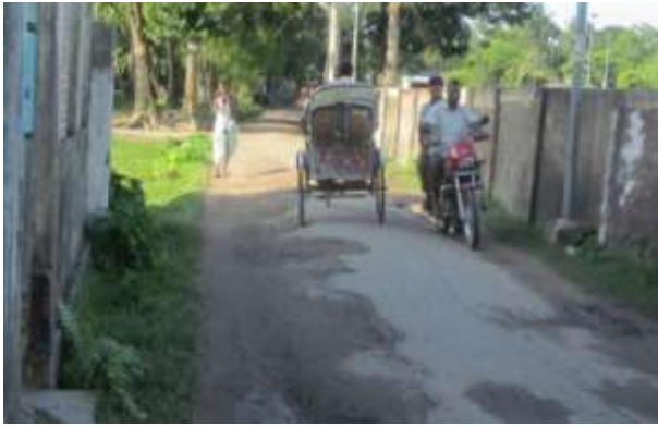
Pourashava road and drain with very badly damaged surface and displaying poor maintenance
