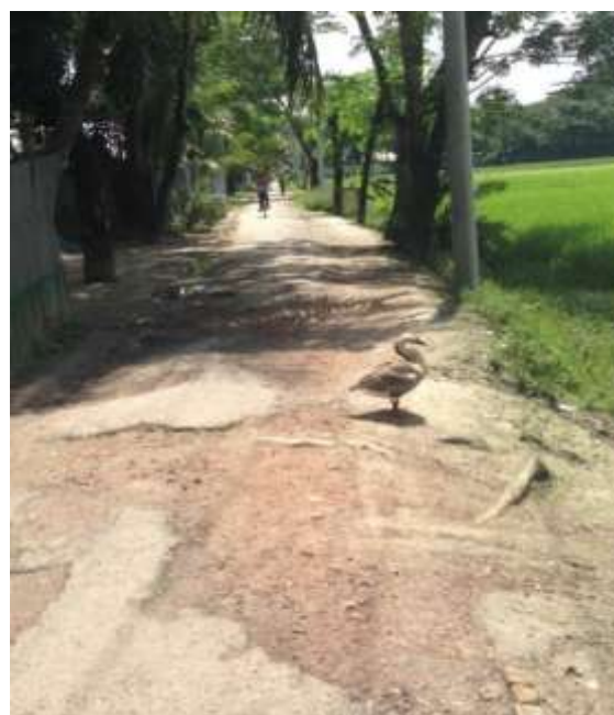
Pourashava road and drain with very badly damaged surface and displaying poor maintenance
