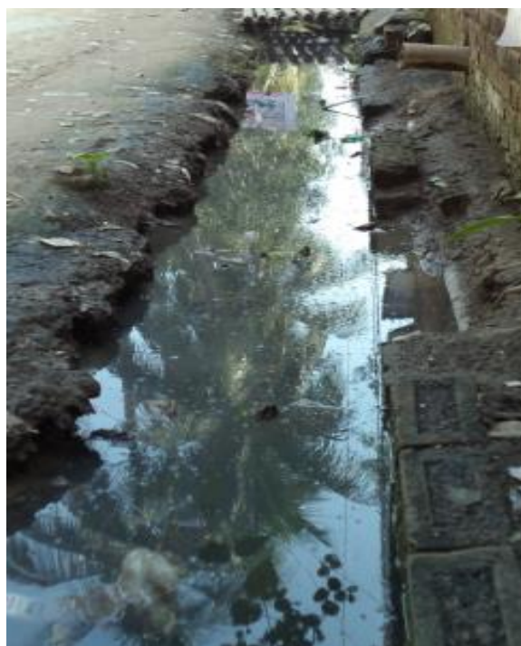
Badly damaged Pourashava roads and drains displaying poor maintenance
