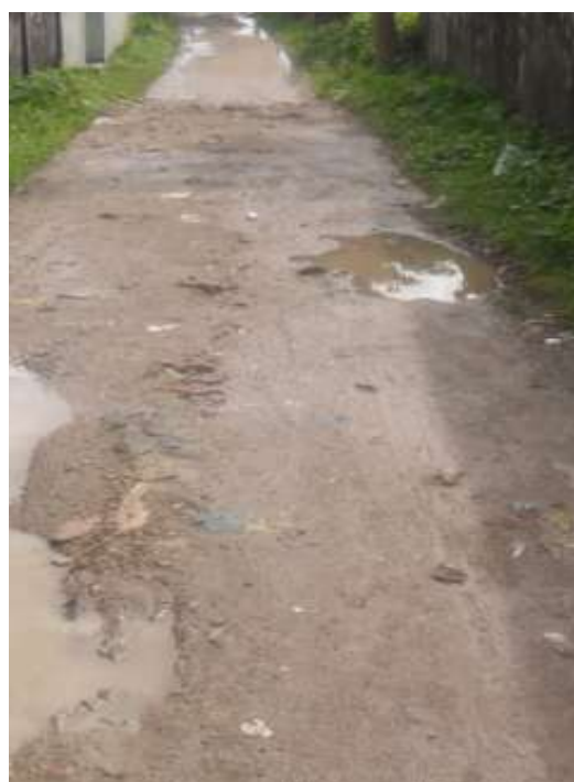
Pourashava road with badly damaged surface and displaying poor maintenance
