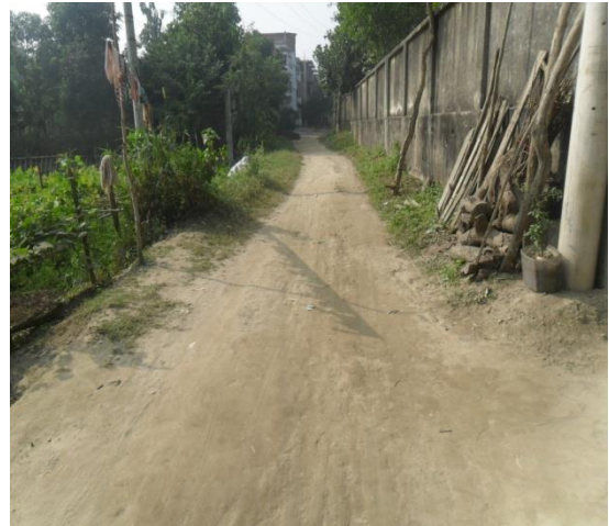
Proposed road and road side drain with very badly damaged surface and displaying poor maintenance
