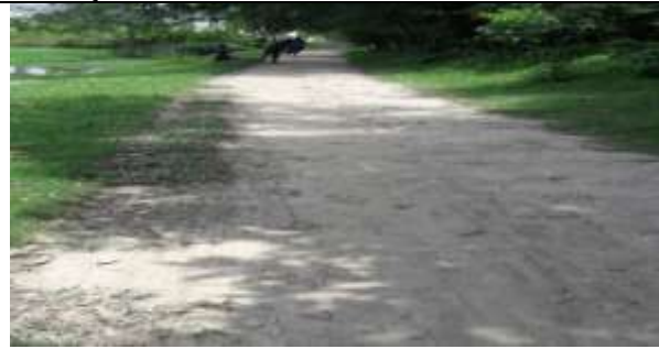
P-17(PDP-TLCC): Construction of road from volachang Gunin para H/O Aziz Mia to Shuhata LGED road via Valanagar Bridge by CC. Ch 0.00-917.00m and Connecting road from Jamal Mia House to Debu Thakur House via H/O Kamal Mia by CC. Ch 0.00-300.00m
