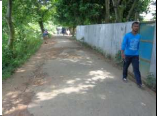
P-08(PDP-TLCC): Construction & widening of road from Nabinagar Eichhamoye girls school to Alamnagar uttarpara by CC. ch. 0.00-1150.00m
