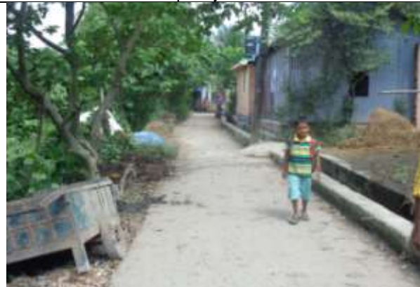
P-15 (PDP-16): Construction & widening of Alamnagar Southpara Golam Mostofa House to Alamnagar Northpara Lapang River Road by CC.Ch. 0.00-2242.00m .and Construction of connecting road from Alamnagar Northpara Shanti Kutir to H/O Gulgar Mia Road by CC.ch. 0.00-340.00m.
