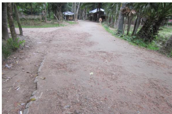
Pourashava road with very badly damaged surface and displaying poor maintenance
