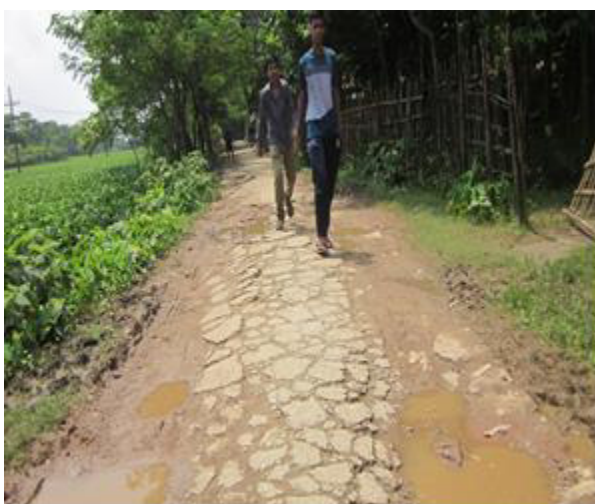
Pourashava road and drain with very badly damaged surface and displaying poor maintenance
