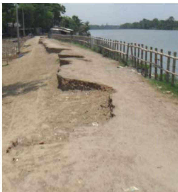
Pourashava – Roads and Drains very badly damaged and displaying poor maintenance
