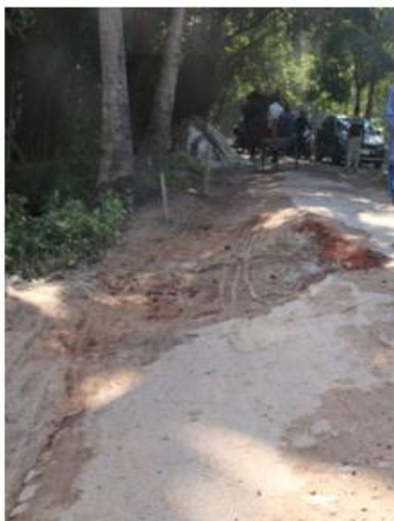
Pourashava roads with badly damaged surface and displaying poor maintenance
