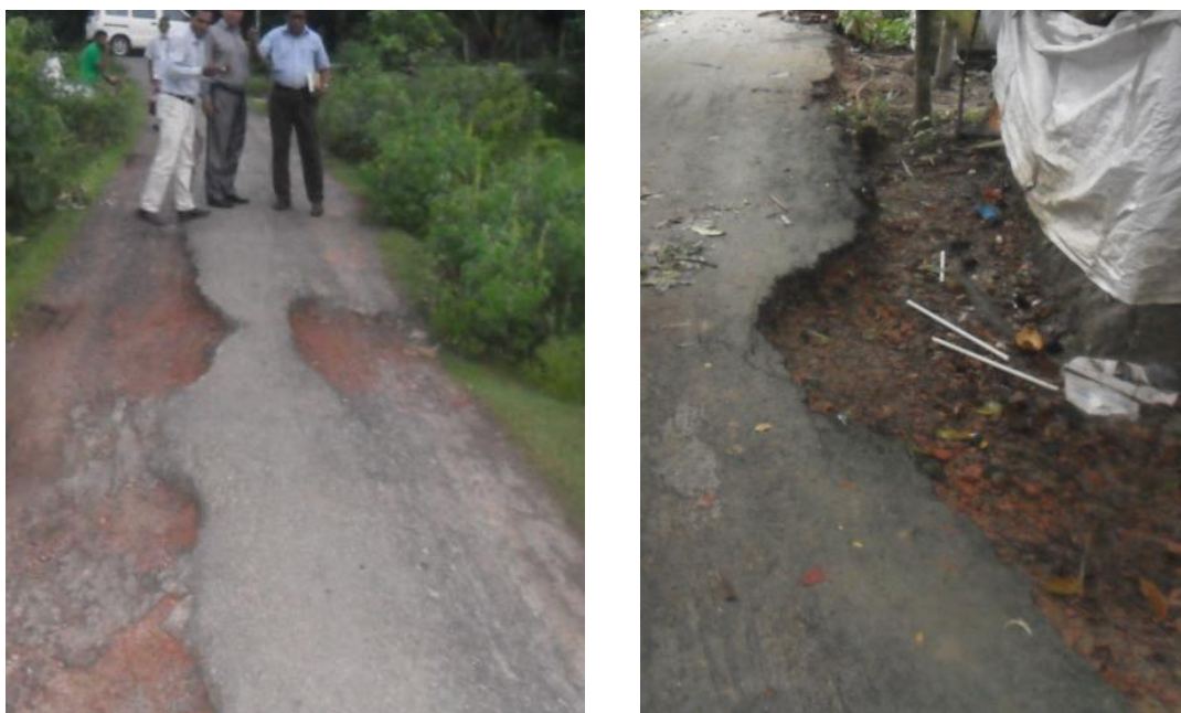
Pourashava road with badly damaged surface and displaying poor maintenance
