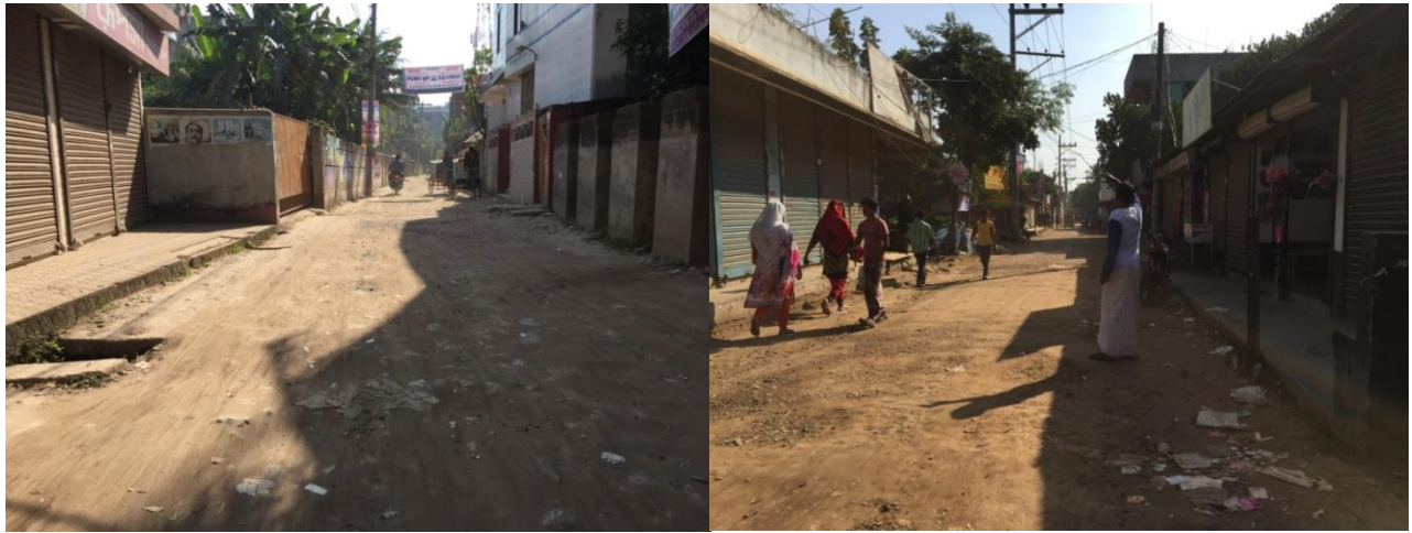
Pourashava road and drain with very badly damaged surface and displaying poor maintenance
