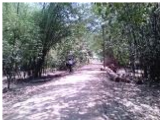
R17: Existing road condition, April 24, 2014
