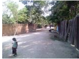
R13: Existing road condition, April 24, 2014
