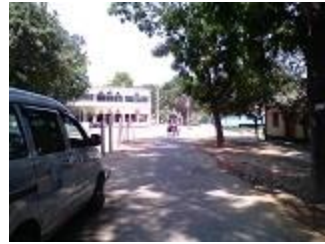
R4: Existing road condition, April 24, 2014
