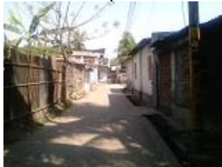
R3: Existing road condition, April 24, 2014
