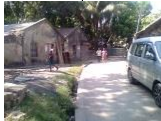
R3: Existing road condition, April 24, 2014
