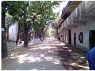
R4: Existing road condition, April 24, 2014
