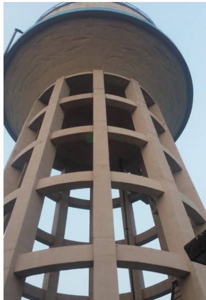
Figure 3: Existing Overhead Tank in Joypurhat Pourashava
