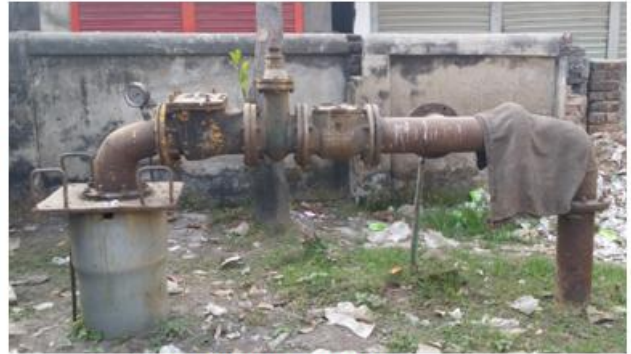
Existing Production Tube well Site
