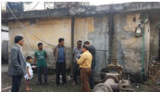
Data Collection & Visit – existing Water Supply Site
