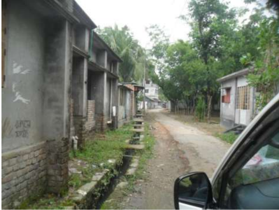
Existing Katchha Drain proposed for R.C.C. construction
