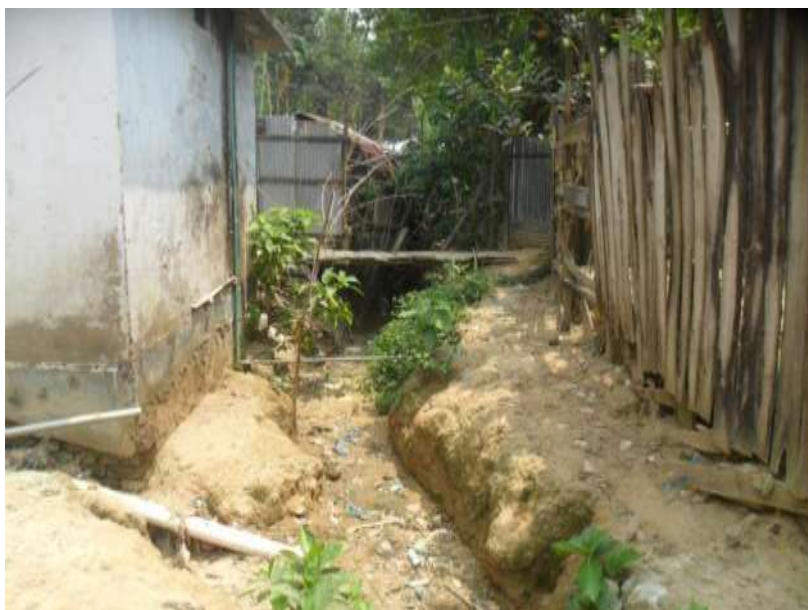
Existing Katchha Drain proposed for R.C.C. construction
