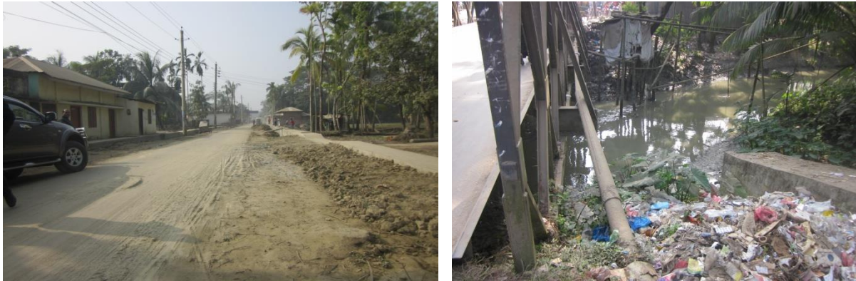
Pourashava road and drain with very badly damaged surface and displaying poor maintenance
