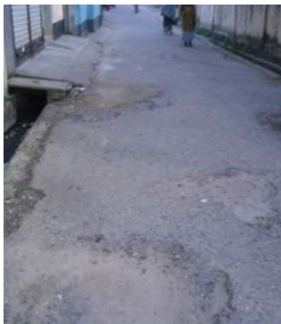
Pourashava road with very badly damaged surface and displaying poor maintenance
