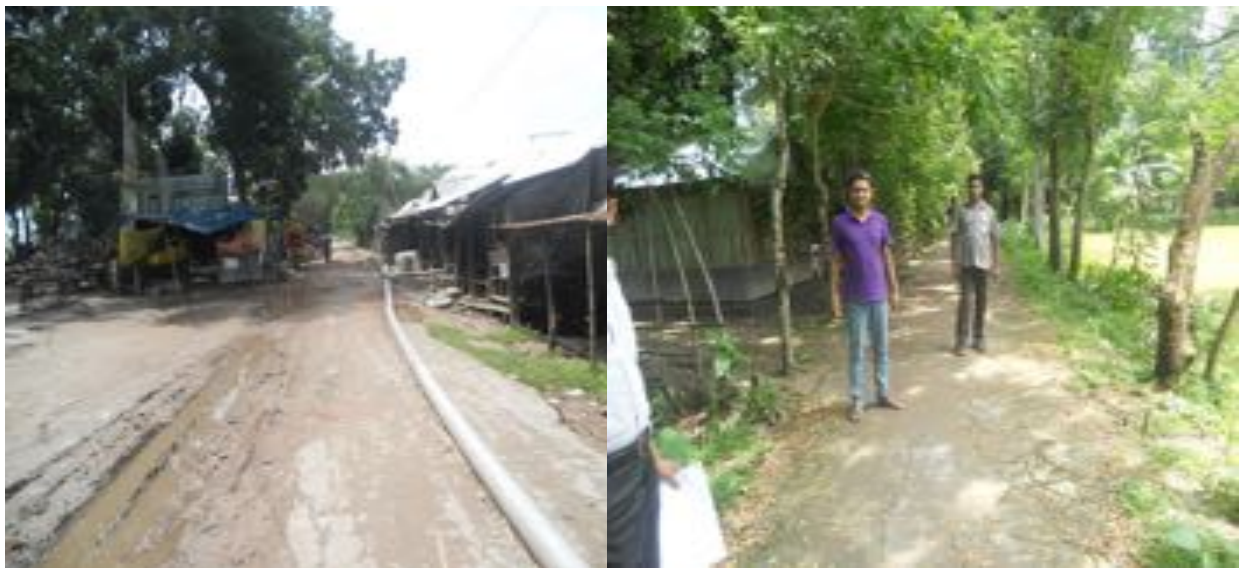
Pourashava road and drain with very badly damaged surface and displaying poor maintenance
