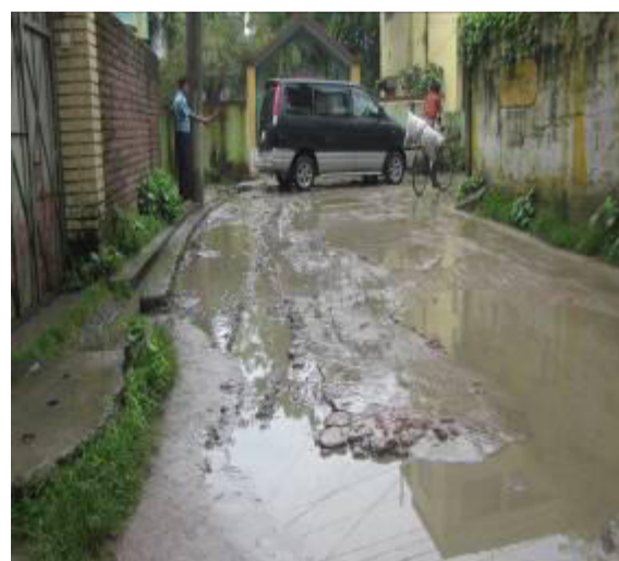
Pourashava road and drain with very badly damaged surface and displaying poor maintenance
