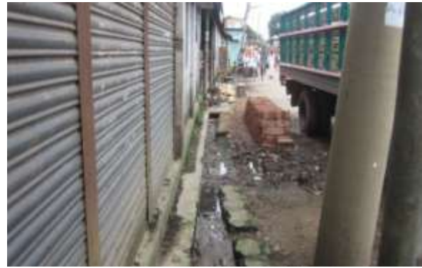
Pourashava road and drain with very badly damaged condition and displaying poor maintenance
