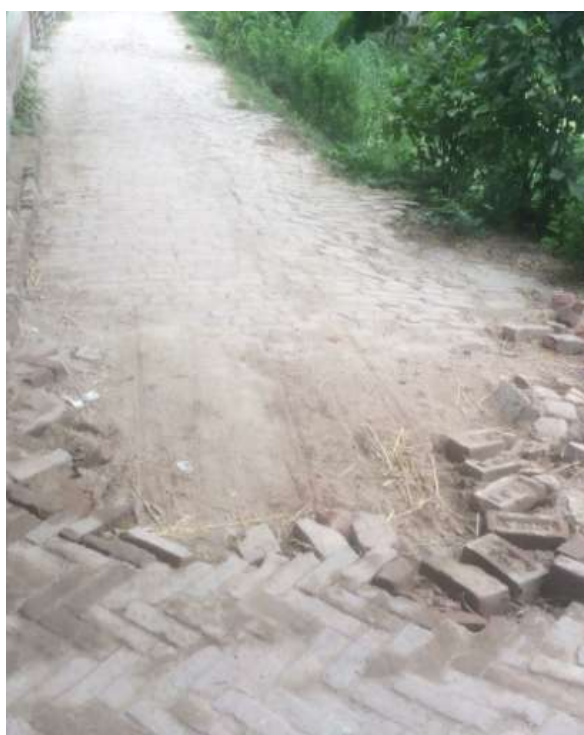
Pourashava road and drain with badly damaged surface and displaying poor maintenance
