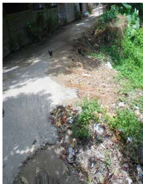
Pourashava road and drain with badly damaged surface and displaying poor maintenance
