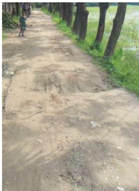
Pourashava road with badly damaged surface and displaying poor condition
