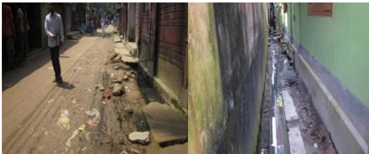
Pourashava road and drain with very badly damaged surface and displaying poor maintenance
