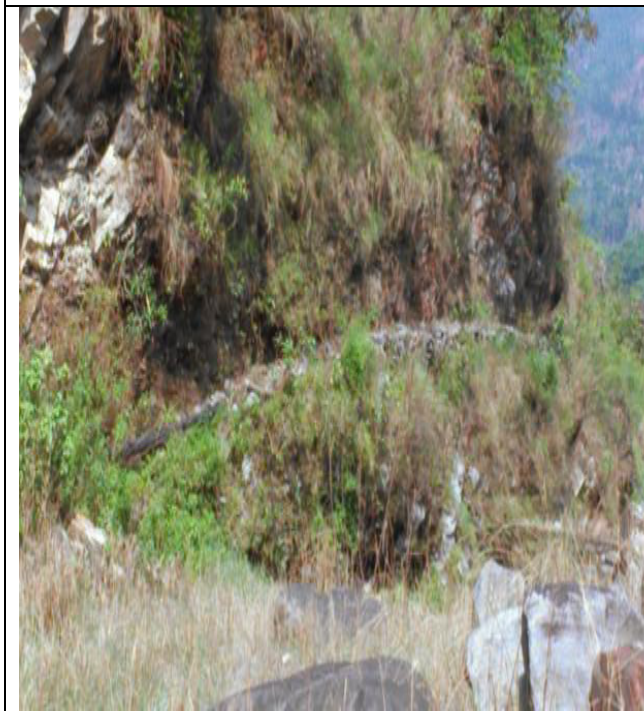
Existing transmission main from Ritha Ghari, Phalakhu river, Gerku VDC
