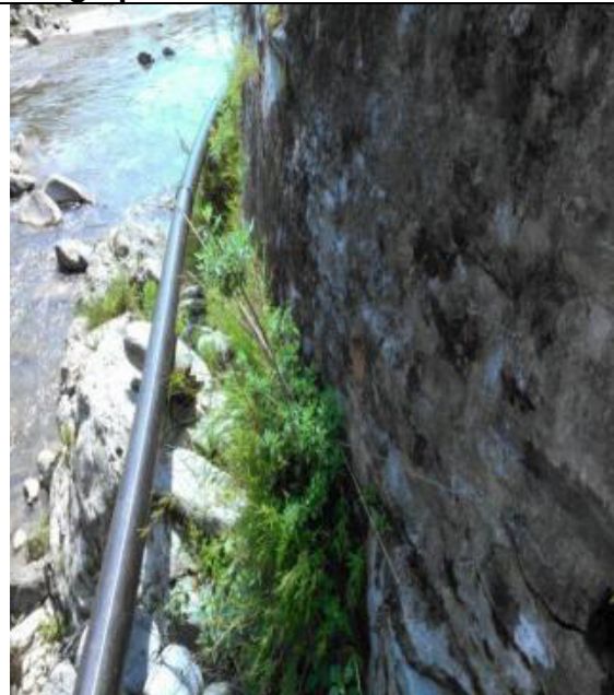
Transmission main from Phalakhu river to Bidur Treatment plant through very difficult terrain
