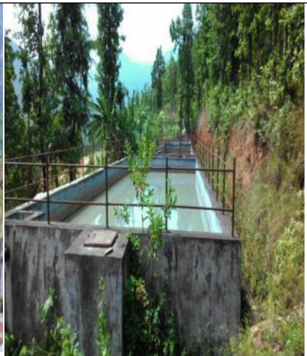
Existing reservoir tank at ward no 3, Bidur Municipality
