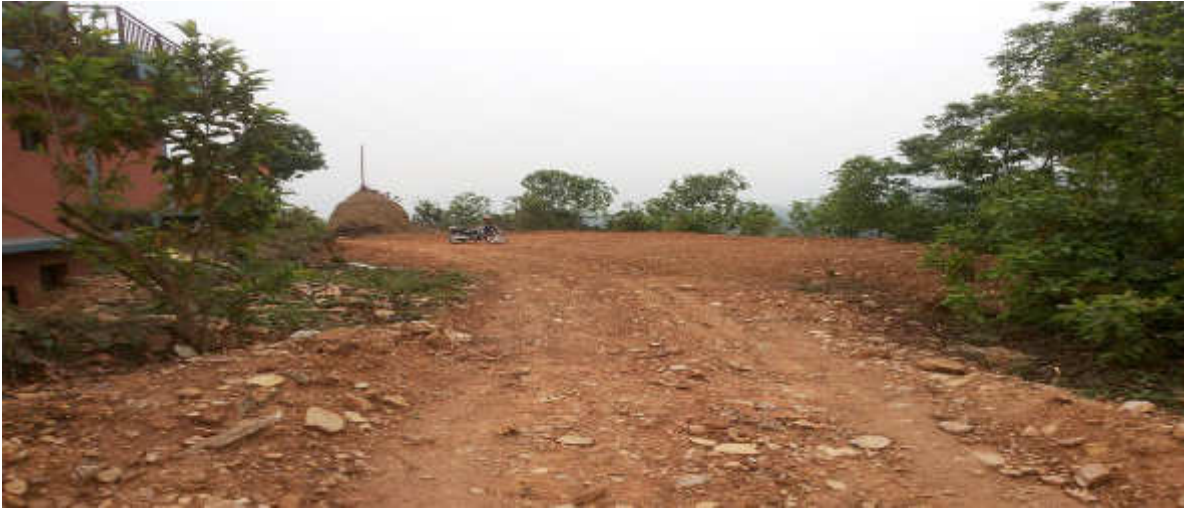
Figure 1 Recently Acquired Land for RVT -Paite
