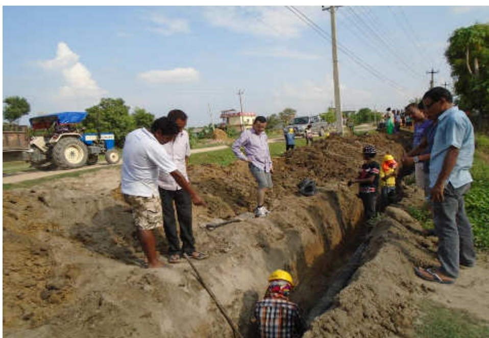
DI Pipe laying works, Tikapur, Kailali
