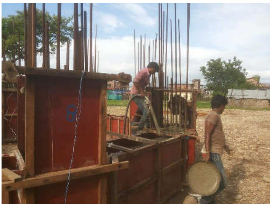
OHT, Bracing beam casting Block 19, Tikapur, Kailali
