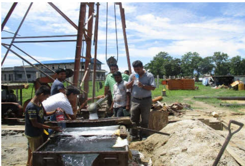
Deep Well, Block 19, Discharge-30 lps, Tikapur, Kailali
