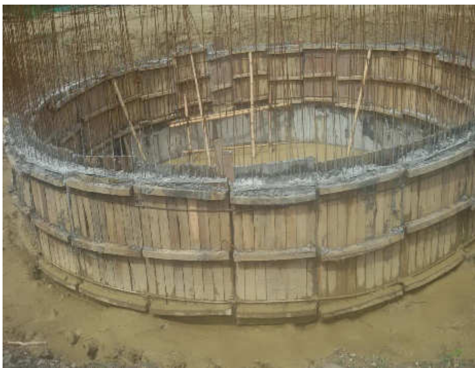
3 rd Lift of RVT Shear Wall at Existing OHT Site, Mirchaiya, Siraha
