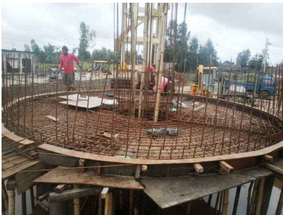
Slab Casting for Filter Medial Placing, Sakhuwa MahendraNagar, Dhanusha
