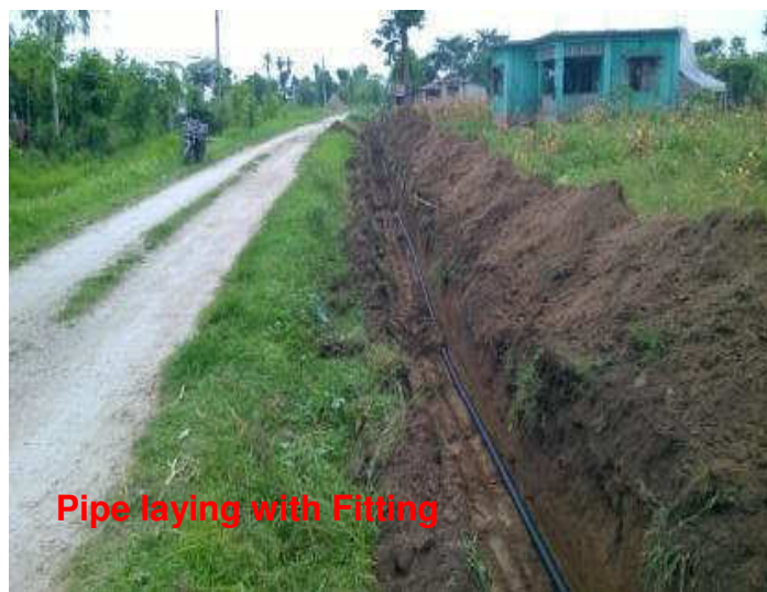
Excavation for Pipe Laying
