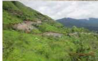
Access Road constructed by DDC to Proposed Dumping site, at the same location DDC/VDC have provided the land for construction of sludge drying bed for septage management.
