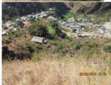
3- RVT-3 & Treatment Plant-2
