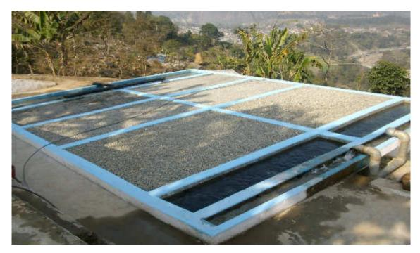
Existing Roughing Filter and Proposed Roughing Filter Site
