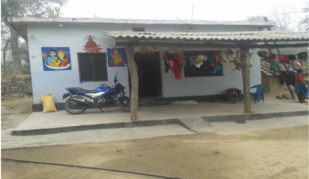
House of Affected Family (Kalawoti Devi Bohara)
