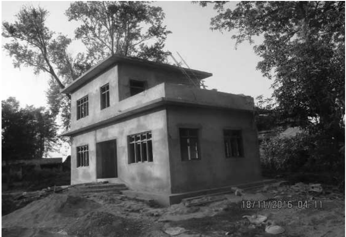
Office Building of Chandrauta, Kapilvastu
