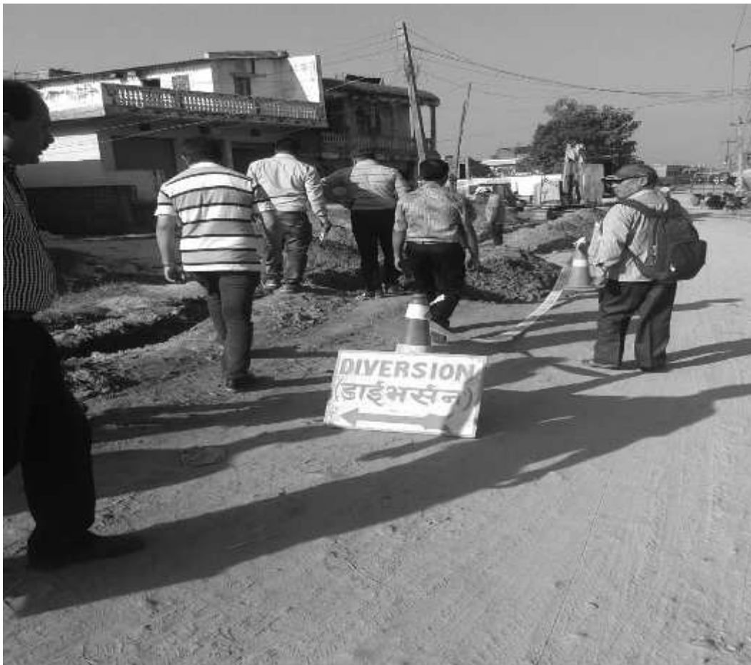
Pipe Laying works Observed by RPMO Engineer, Technical Auditor and Social Safeguard Specialist of DRTAC at Sakhuwa Mahendranagar, Dhanusha
