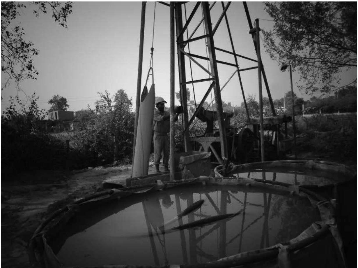
Deep tube well drilling work depth 40m drilling ongoing 4th deep tube well
