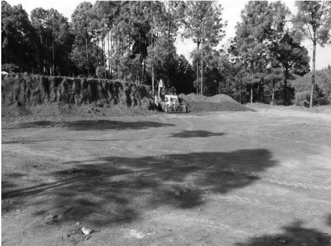
Excavation work continue for 1000 cum Reservoir in Bidur, Nuwakot
