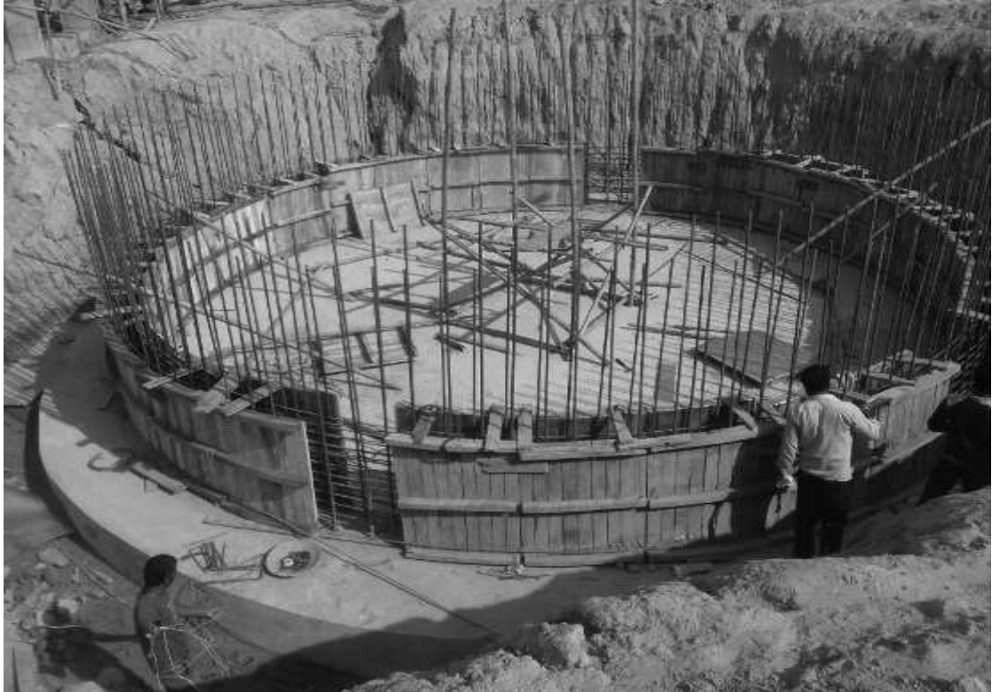
Ground RVT at Matiyarwa site in Mirchaiya, Siraha
