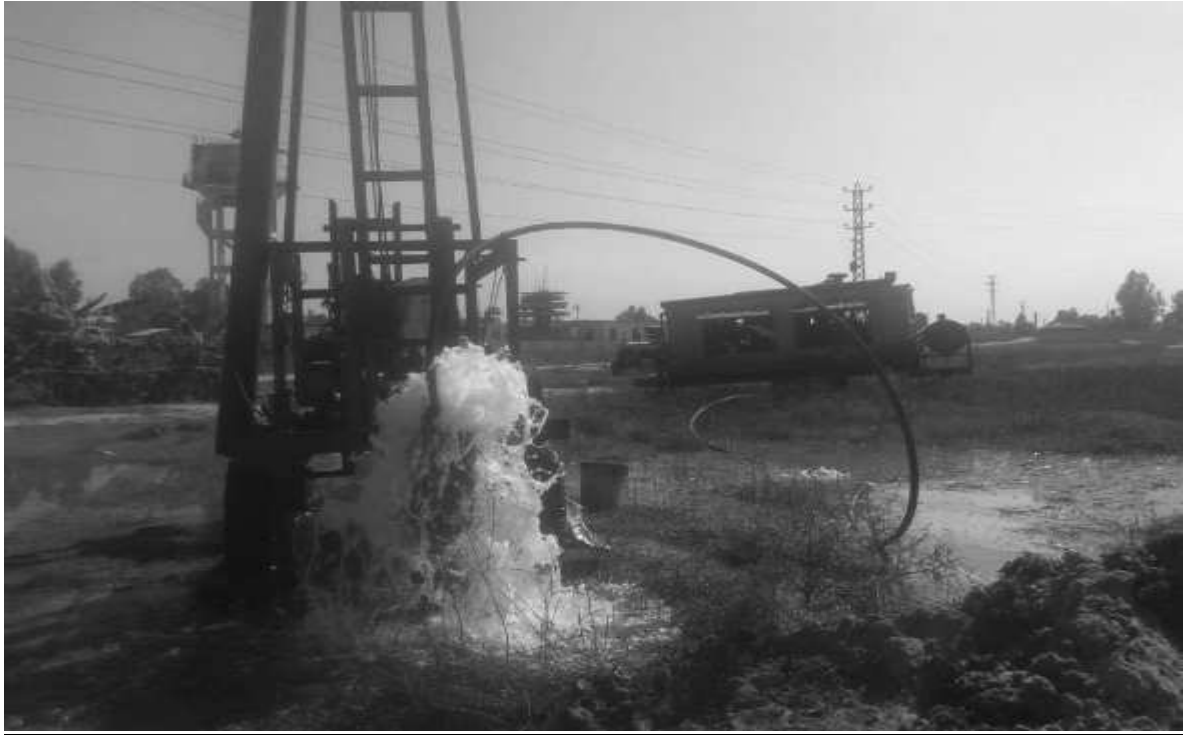
Well development by Air Compressor in Sakhuwa Mahendranagar, Dhanusha
