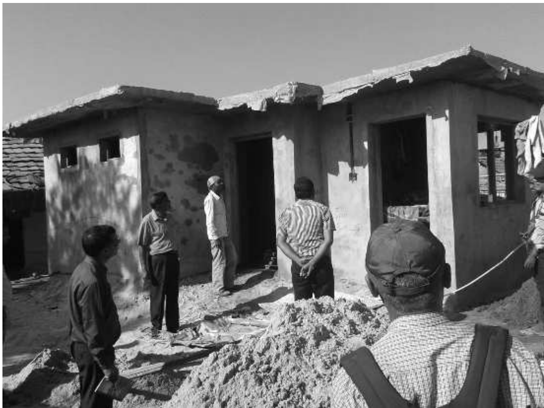
Site Visit of Public Toilet by RPMO, DRTAC and DSMC in Sakhuwa Mahendranagar, Dhanusha
