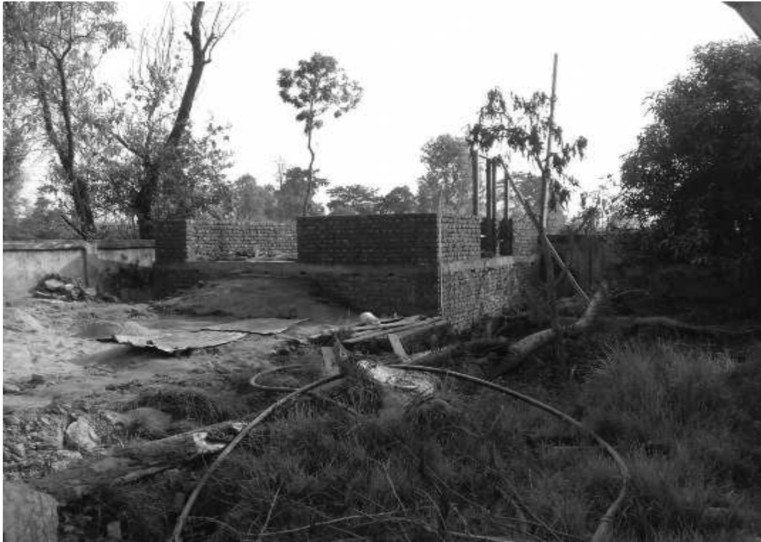
Generator House at existing OHT site in Mirchaiya, Siraha
