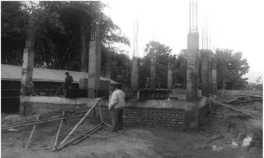
Office Building under Construction of Mahendranagar, Sunsari
