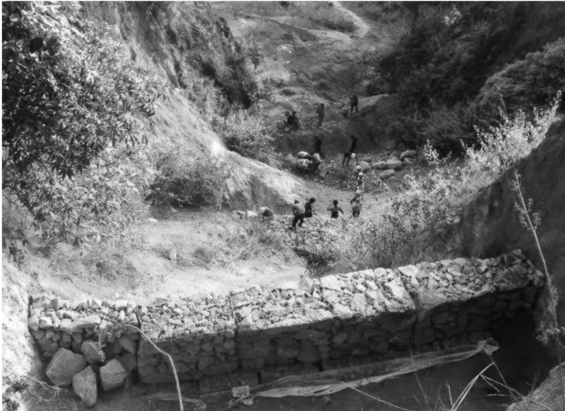
Gabion Protection work at Barahi (Divakar) Danda
