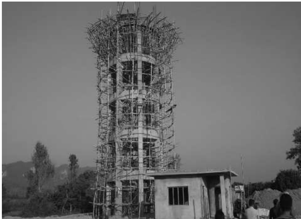
OHT & Guard House at Chhaghariya, Mirchiaya, Siraha
