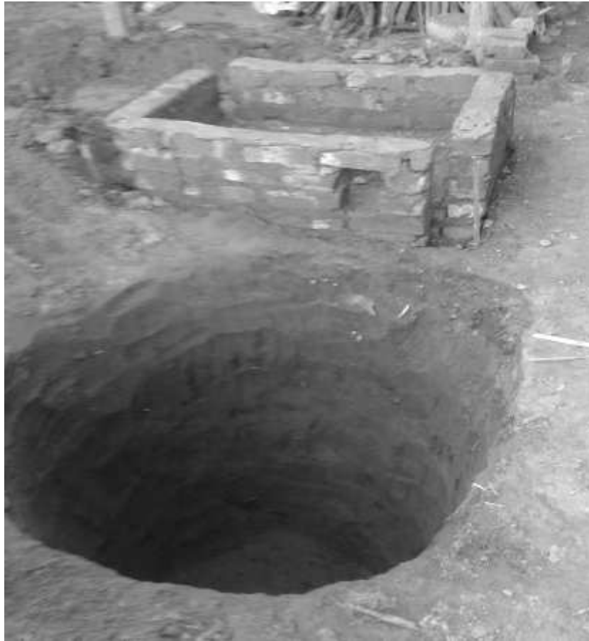
Household Latrines Constructing under OBA Program, Mirchaiya
