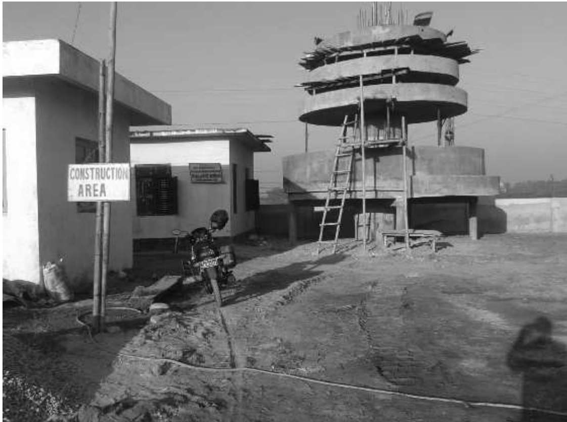
Latest Construction Works in Sakhuwa Mahendranagar, Dhanusha
