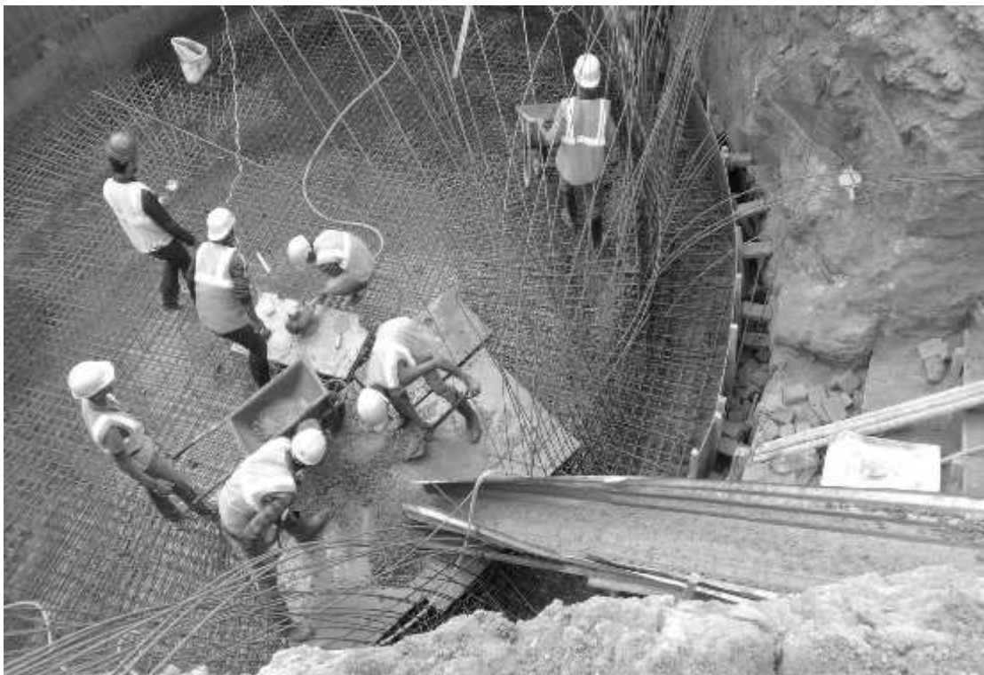
RCC work for Underground Reservoir Tank at Dumre, Tanahu
