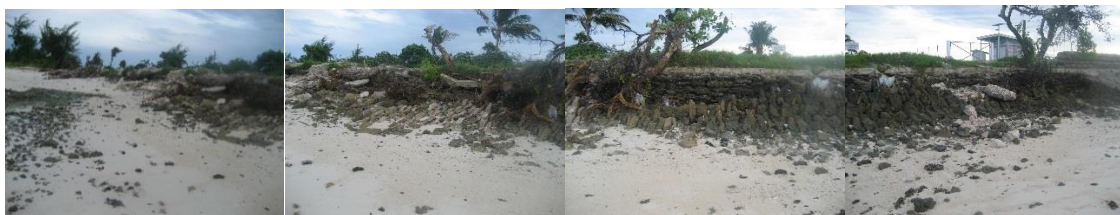
Site 2 works area showing broken seawall. Remaining seawall is visible in right hand photograph.
