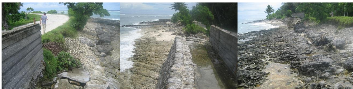
Site 11: existing coastal protection works and nearby habitats
