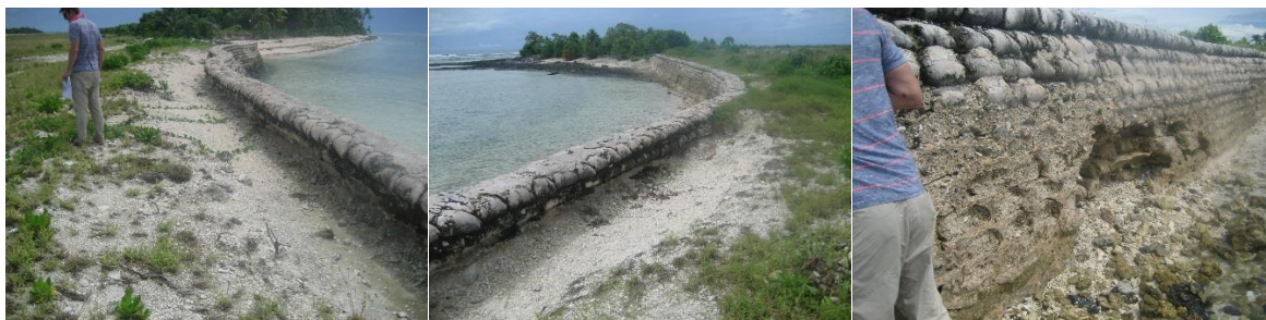
Views of the existing seawall and foreshore at Site 15N
