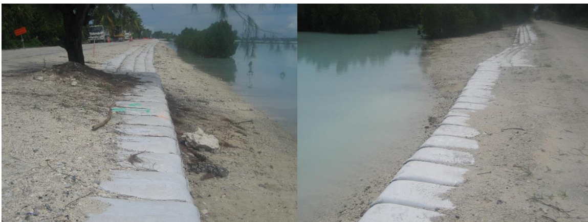
Coastal protection works on the Ananau Causeway
