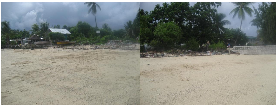
Site 6 – KAP-II seawall visible at right, informal rock wall visible at left.
