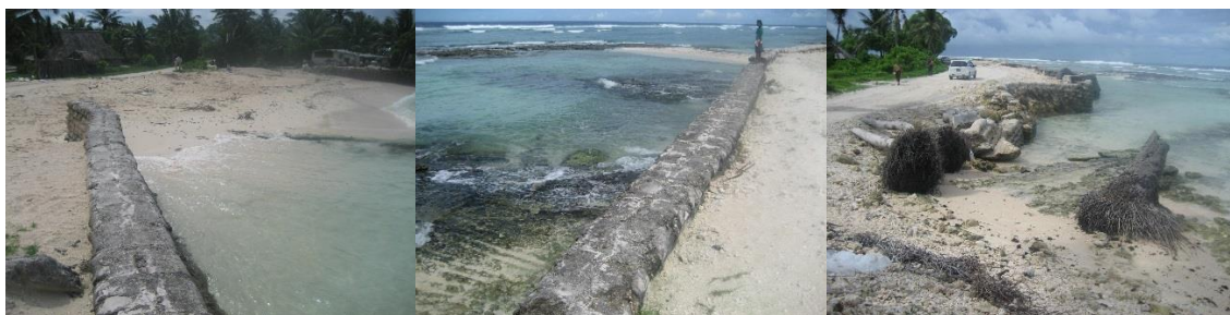
Site 10: Eastern end (outflanking); central section; western end (seawall failure)
