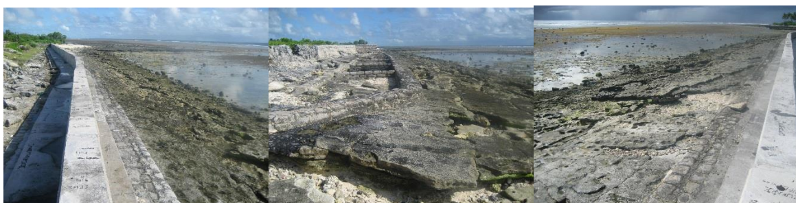
Views of the existing seawall and foreshore at Site 15E
