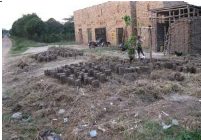
Plate 3.9 Brick laying to support sprouting rural growth centres
