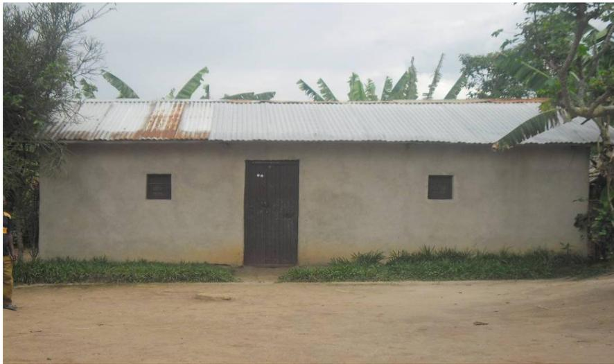
**Figure 3: Iron sheet roofed dwelling unit with temporal walling**
