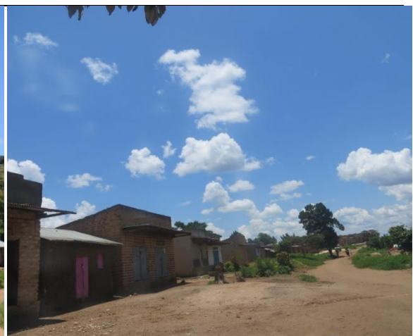
Figure 17: Linear Structures at Kirumbi RGC
