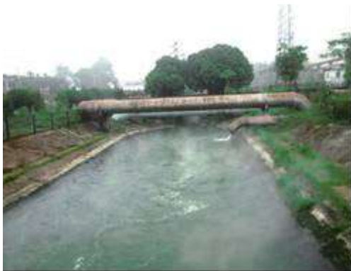
Photo 6-1: Condenser cooling water discharge canal
