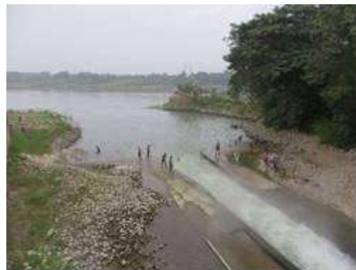
Photo 6-2: Condenser cooling water outfall at Palash Bazar
